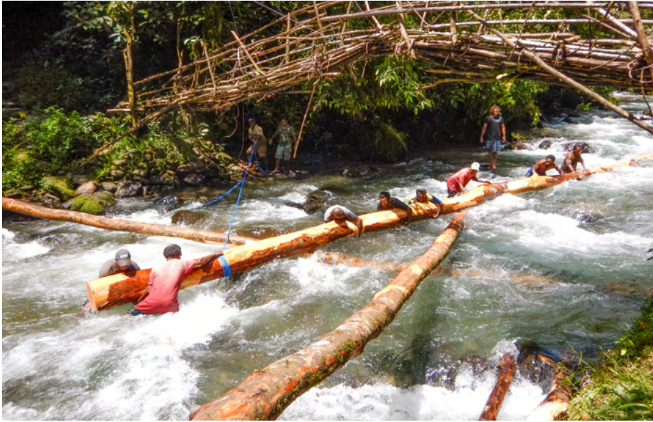
Community members from Manari village carry a log across Emuni creek to build a new bridge
