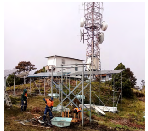
Upgrade of radios at Mt Fala
